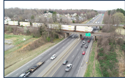
NSR MAINLINE ADJACENT TO GROVES ST.
